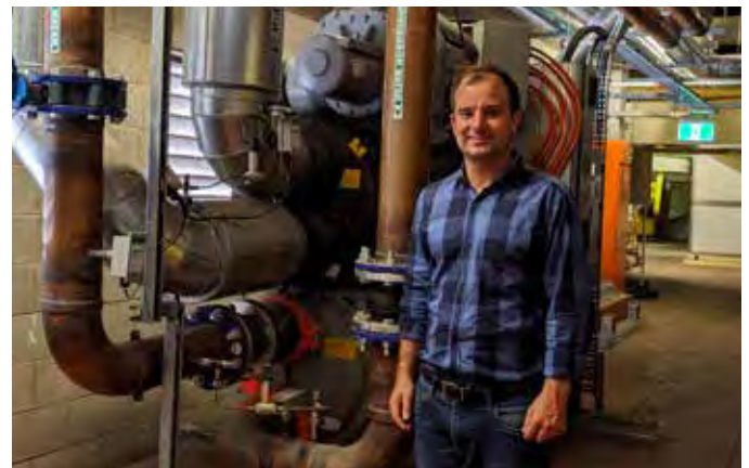
The sustainability features of a new chiller system in Centre Block of The Alfred, including reduced electricity and water use. Pictured is Tom O'Brien from Engineering Services.
